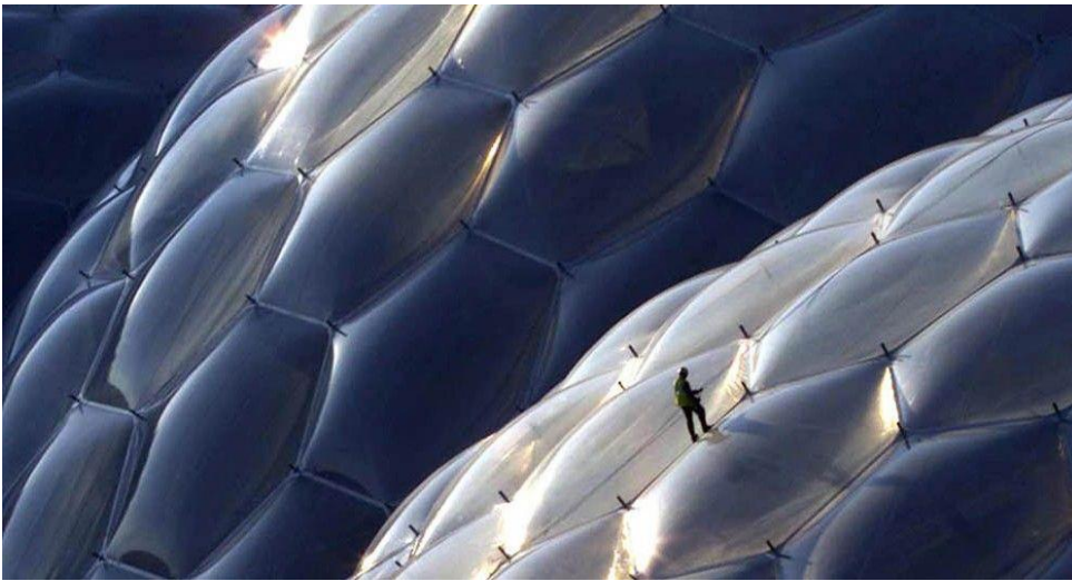
Figure 6. polymer material "ETFE" membrane
