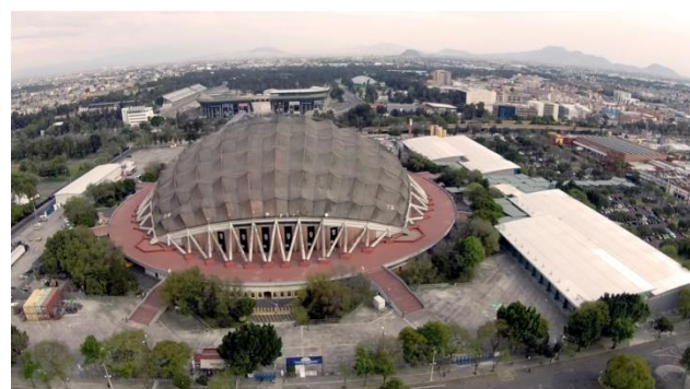
Figure 4. Sports palace in Mexico
