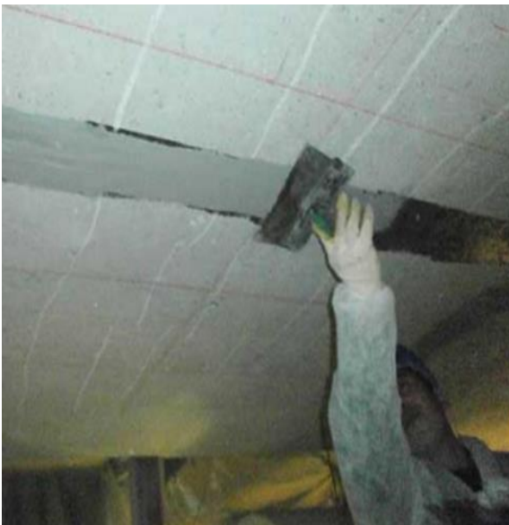
Figure 2. Bonding process of carbon fiber fabric
