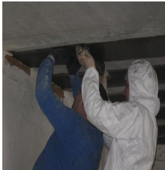
Figure 2. Bonding process of carbon fiber fabric
