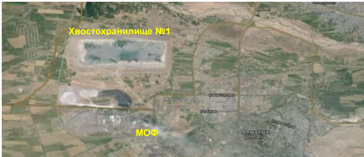
Figure 1. A view of the MOF landfill
